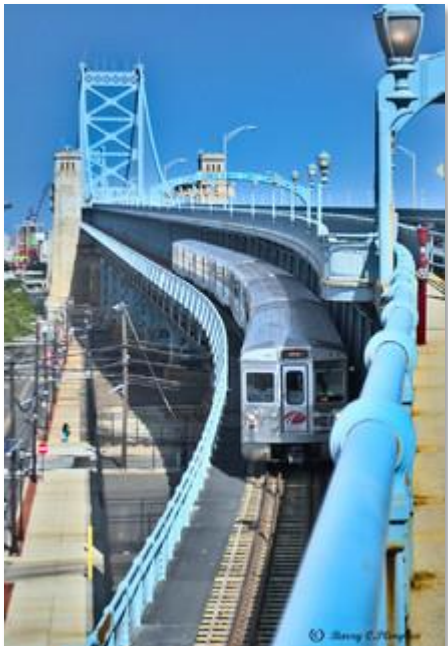
Ben Franklin Bridge Tower - Barry Plimpton
